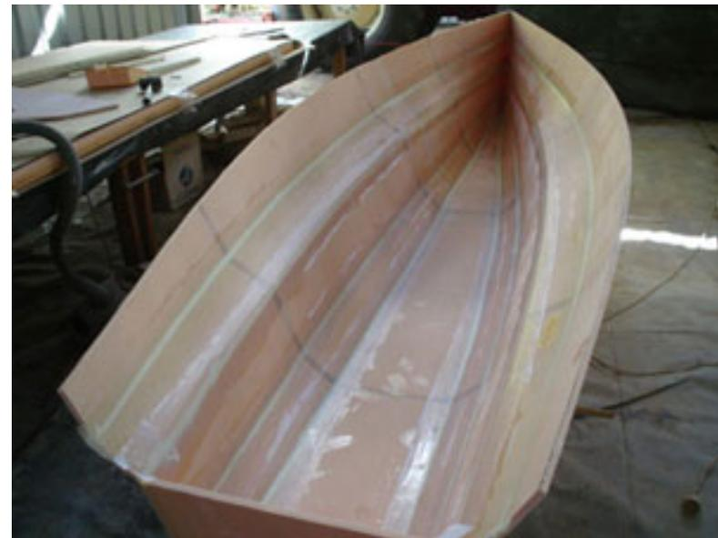
The hull was turned and the chines taped. A quick neat technique is to use a wet fillet. The bog is applied in a rough fillet and the glass tape is applied over the wet fillet. Using a compactor, squeeze out air bubbles and shape the fillet wiping off any excess filler.
