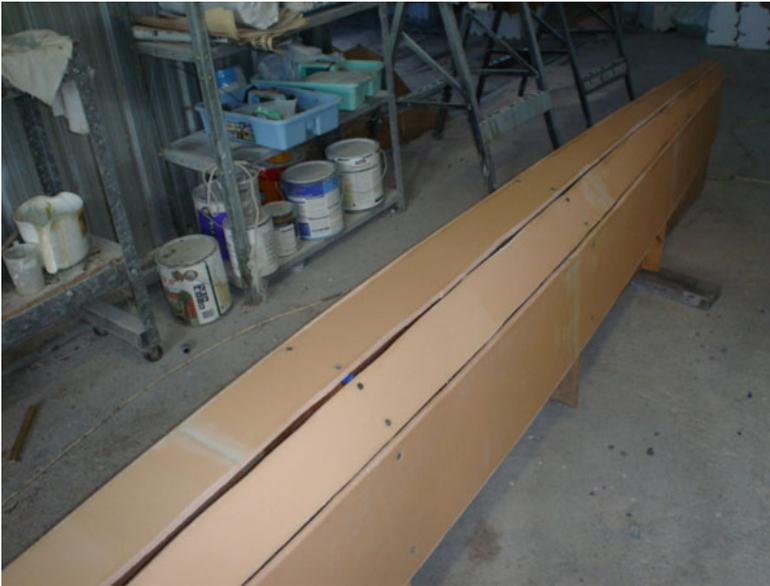
The panels added to the frame and joined with drywall screws (foam) or staples (plywood).
