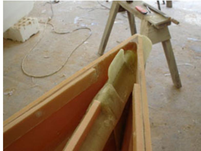
Scrap foam or plywood is glued to the inside of the hull to support the deck. Deck is glassed, trimmed and glued to the supports using soft metal.
